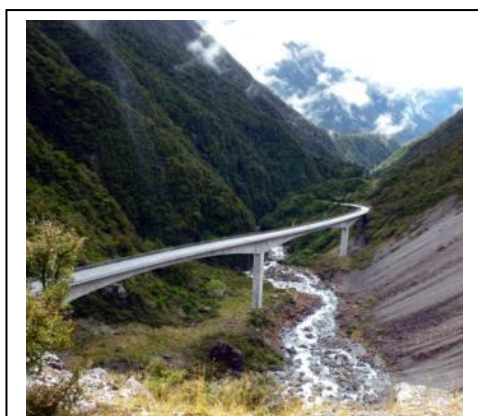
Viaduct through Arthur's Pass
